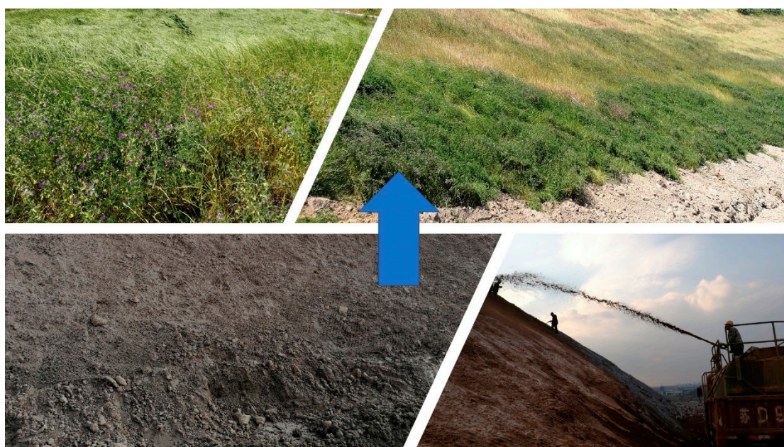
Figure 1. External-soil spray seeding (ESSS) technique.
