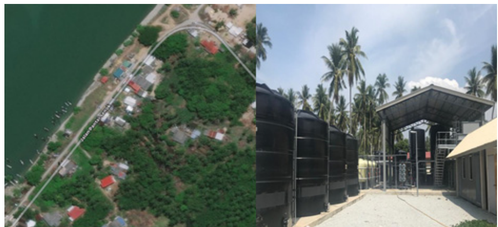
Figure 1. Map of seawater reverse osmosis (SWRO) desalination plant located in Kampung Pantai Senok, Kelantan.
