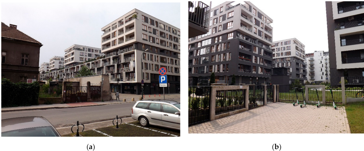
Figure 19. Zabłocie- selected housing projects—as seen in 2020. Photo by authors. (a) difference of scale and density between existing and new architecture; (b) internal green courtyards are accessible only for the inhabitants.
