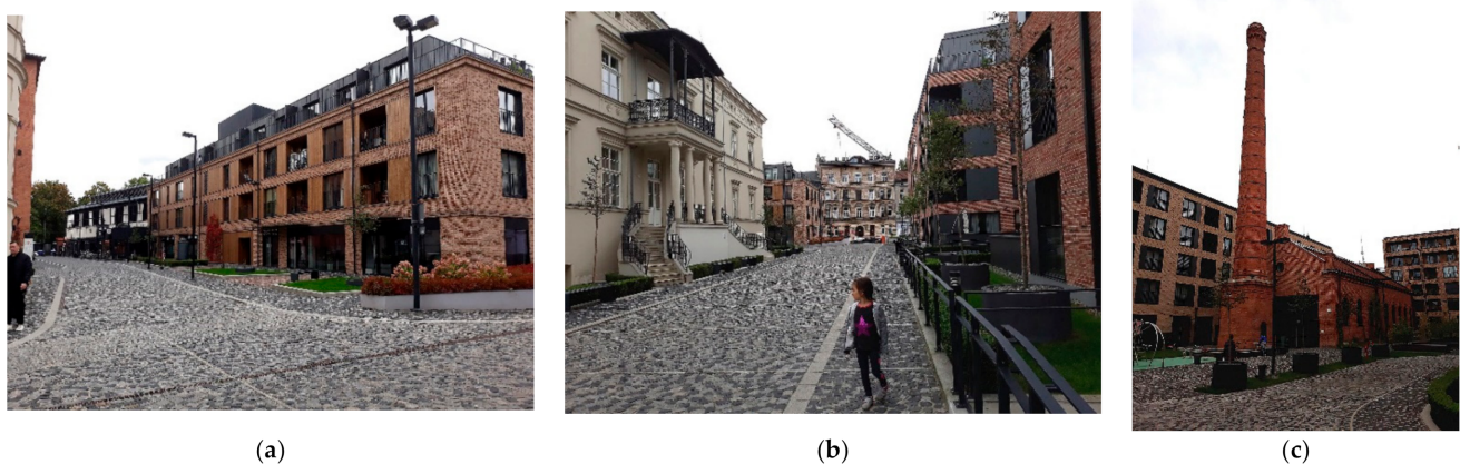
Figure 8. Browar Lubicz housing complex—as seen in 2019. Photo by M.Gyurkovich (a) view from the complex towards the park; (b) internal street with the former palace of the brewery owner on the left; (c) chimney left as a symbol.
