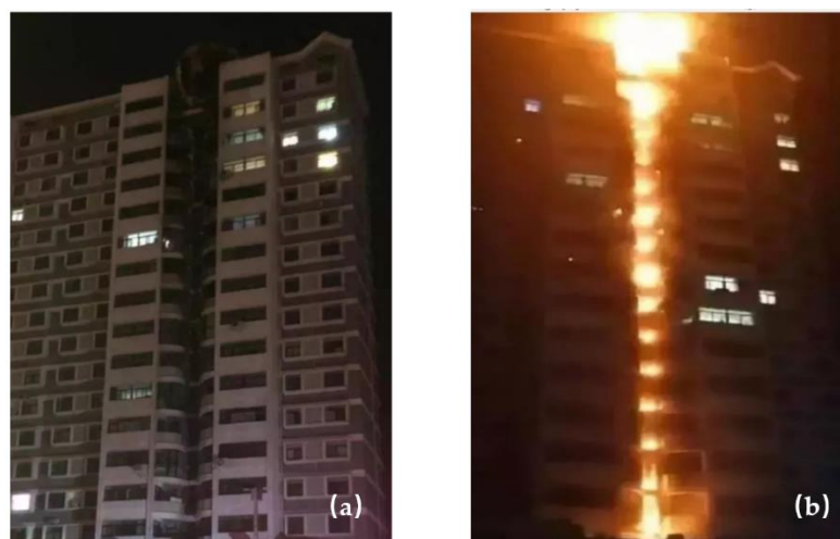
Figure 1. (a) Concave structure of a building; (b) a fire occurring in the concave structure.
